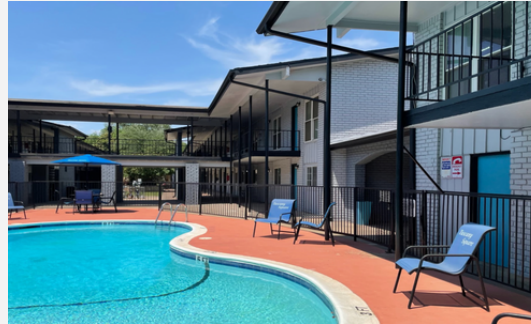
Tuscany Apartments, a 70-unit, Class C garden-style apartment building located in Arlington, Texas
