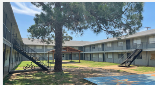
Avalon Apartments, a 75-unit, Class C garden-style apartment building located in Arlington, Texas
